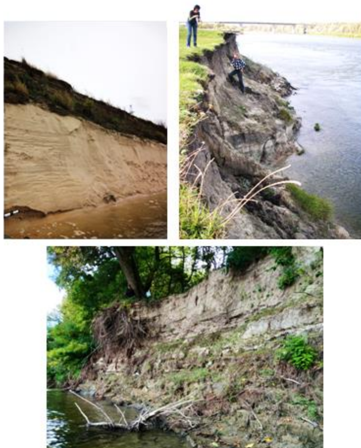
Fig. 2. Steep and landslide-prone banks of the Desna river
